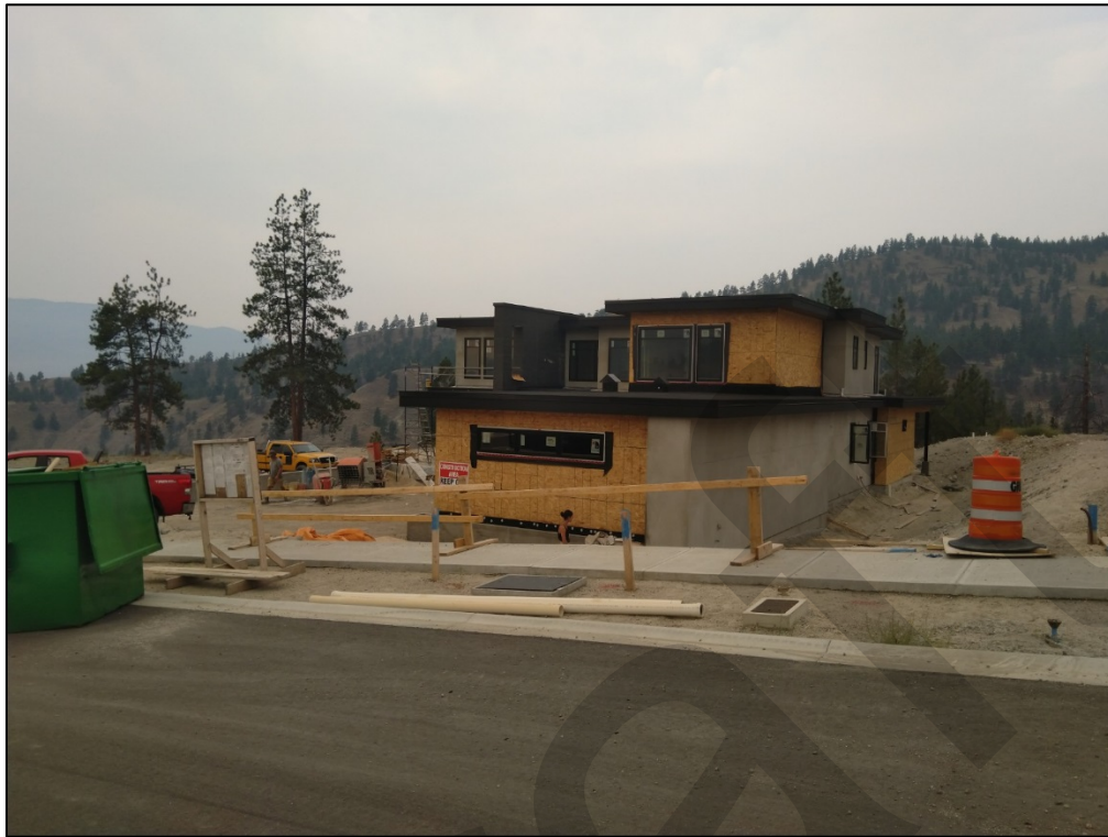
Figure 4: South Elevation showing dwelling under construction
