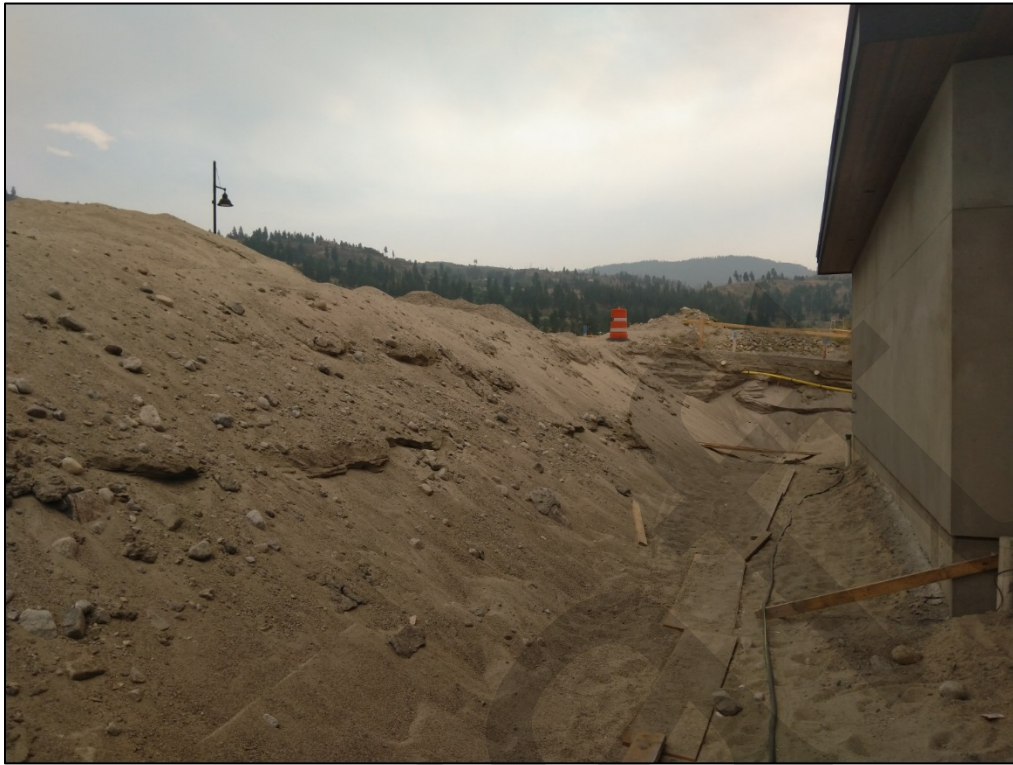
Figure 8: Looking South along east property line
